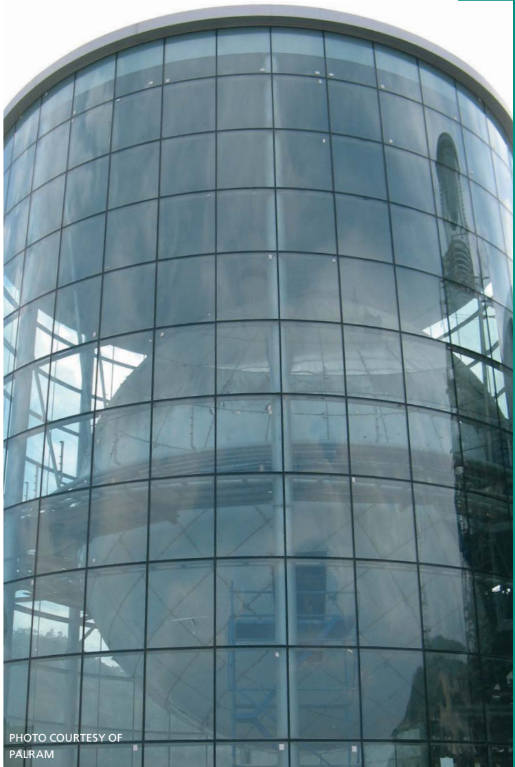
CURTAIN WALLING AROUND ROTATING RESTAURANT
